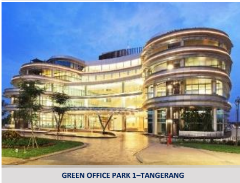
GREEN OFFICE PARK 1–TANGERANG
