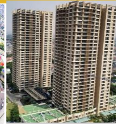
PONDOK INDAH RESIDENCE – JAKARTA
