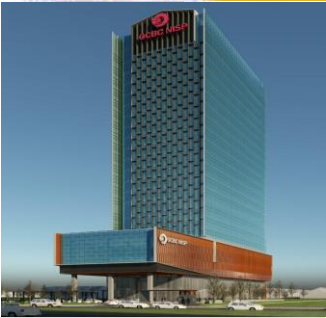
One Tower - BSD City Tangerang
